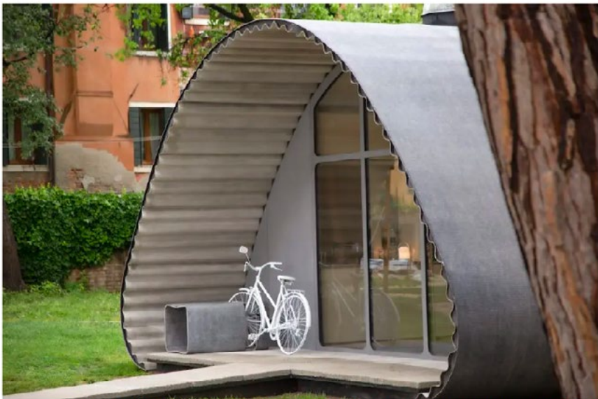
The resilient structure endorses a catenary shape, with low-carbon rollable concrete sheets acting as an external shell. Photo by Mika Cartier
