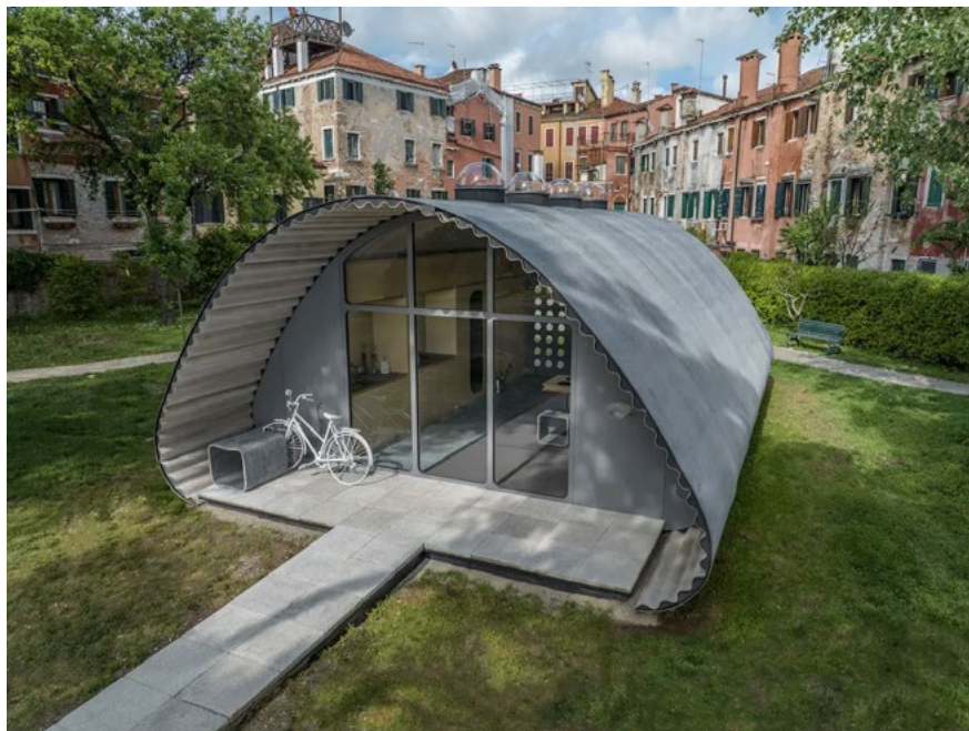
Essential Homes Research Project - @chiarabecattini
