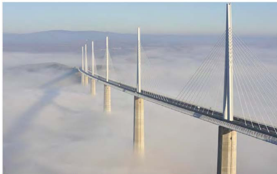
Le Viaduc de Millau, France, designed by Norman Foster CREDIT: Daniel Jamme / Eiffage
